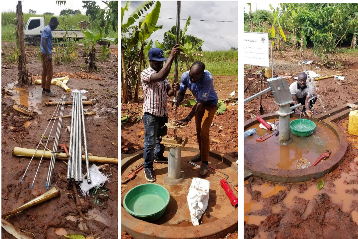
Figure 7: Hand pump installation activities
