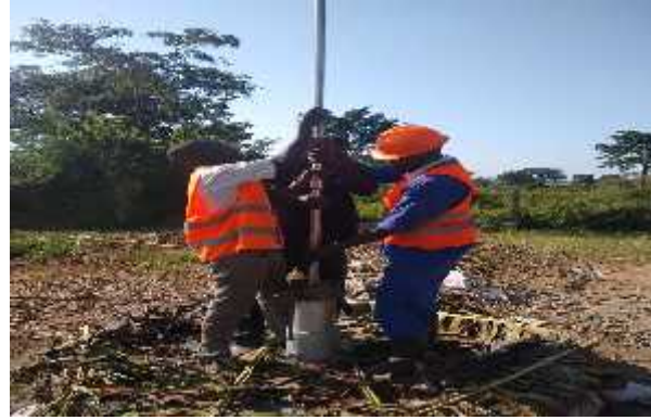
The above photo showing stainless steel pipes and also during Installation in Buyende District
