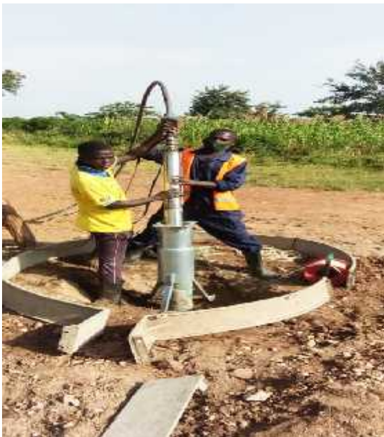
The above photos shows the apron casting, pump testing and a completed borehole.
