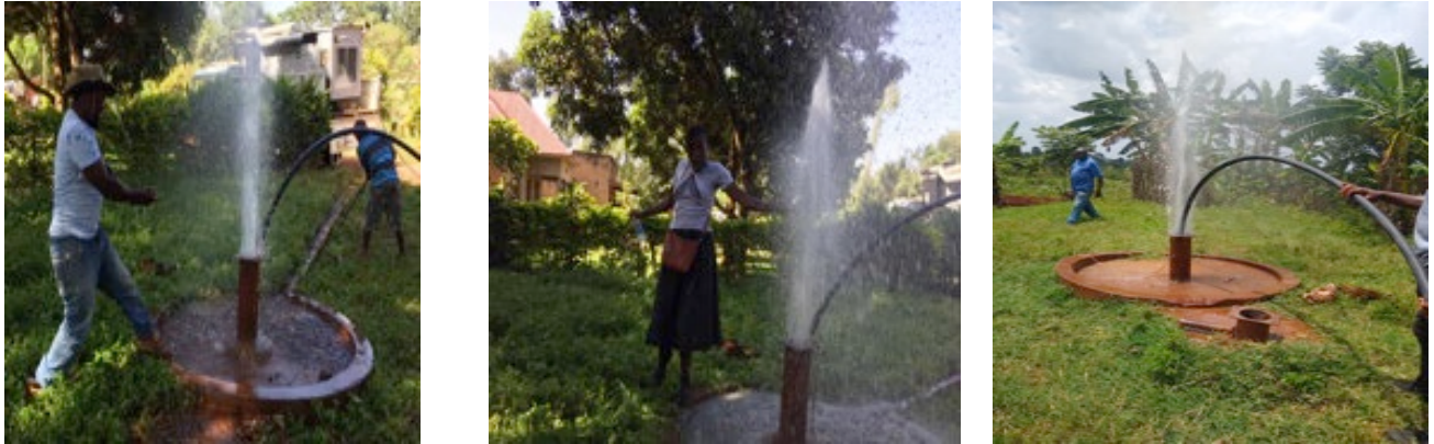
Figure 2: Blowing of Akisofeli, Lwalanda and Musenze boreholes
