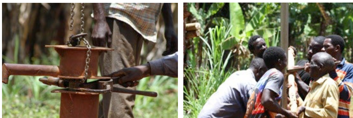
Figure 1: Showing Fishing of Akisofeli borehole
